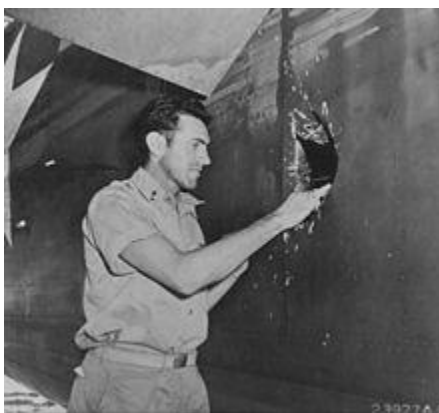
Zamperini examines a hole in his B-24D Liberator Super Man made by a 20 mm shell over Nauru.
